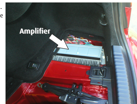
Picture of amplifier in IS250C with boot floor removed
